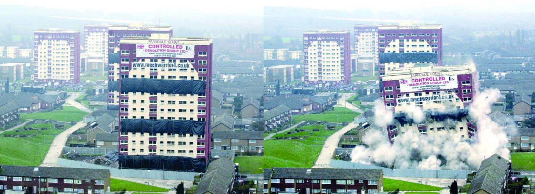
In poor condition and unpopular with tenants, two blocks of flats at Swardcliffe, LS14, were demolished in March 2001.
